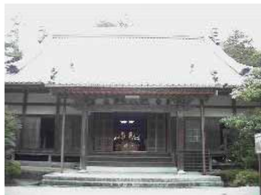
the main building of KOGETSUIN
